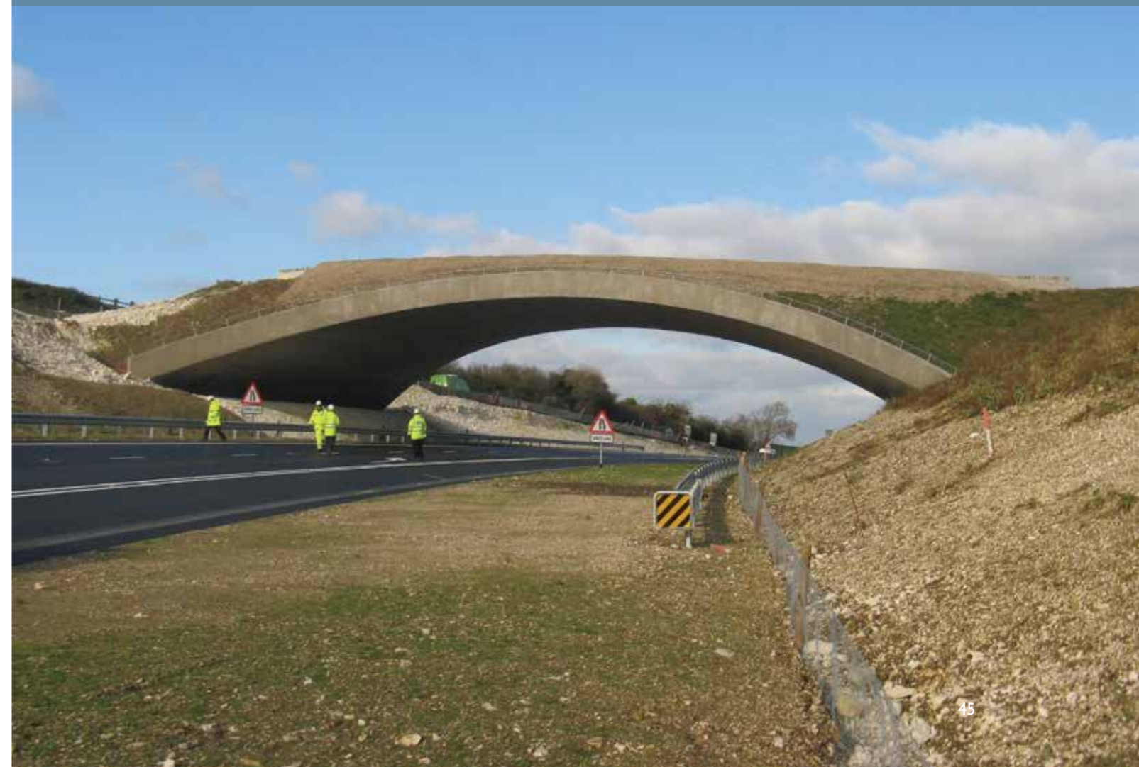
Green bridge over the Weymouth Relief Road
