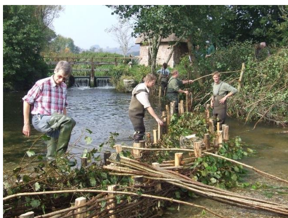
Narrowing the channel after cattle poaching eroded banks Photo: DWT
