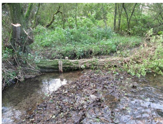
Leaky dams – slowing the peak flow events and 'pushing' the flow out to be held in wet woodland habitats Photo: DWT
