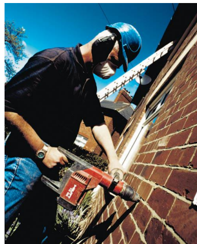
Cavity wall insulation installation Photo: BBC
