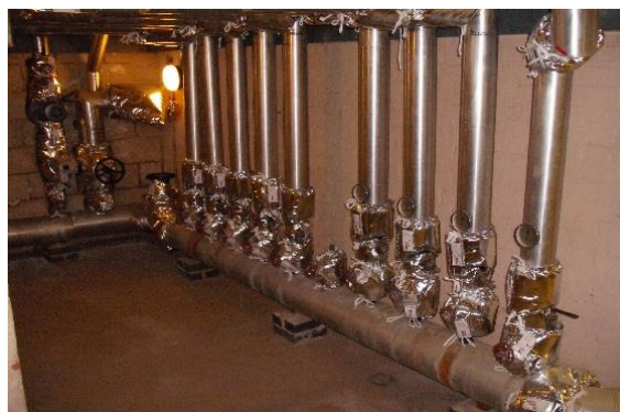
Bournemouth Town Hall boiler room, valve insulation Photo: BBC
