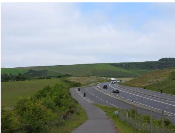
View of the road with the Southdown Ridge road cutting on skyline © John Stobart (NE)
