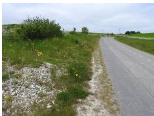
Former road narrowed with flower rich limestone spoil verges © John Stobart (NE)
