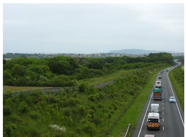
Embanked sound barrier against the Lorton NR. Road aligned to minimise losses to Two Mile Coppice © John Stobart (NE)
